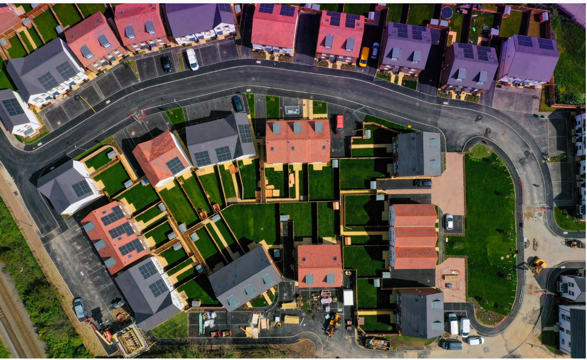
↑ Pictured: Green Vale development, Worcestershire
