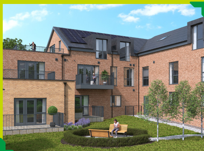
Solar panels at Westcliffs, Southend
