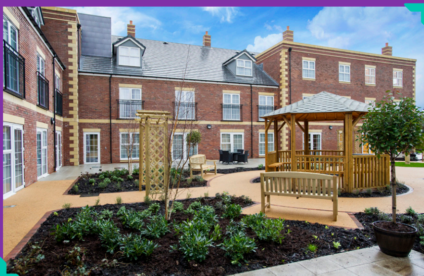
Upton Dene Residential and Nursing Home, Cheshire
